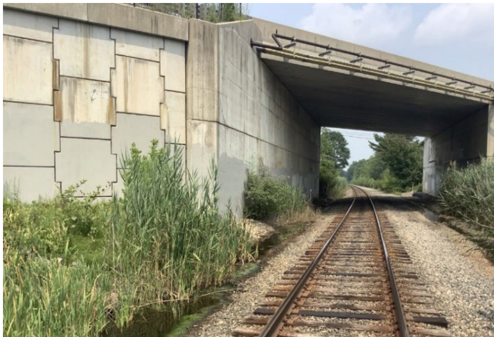
Amtrak Rail Corridor Under Route 111
